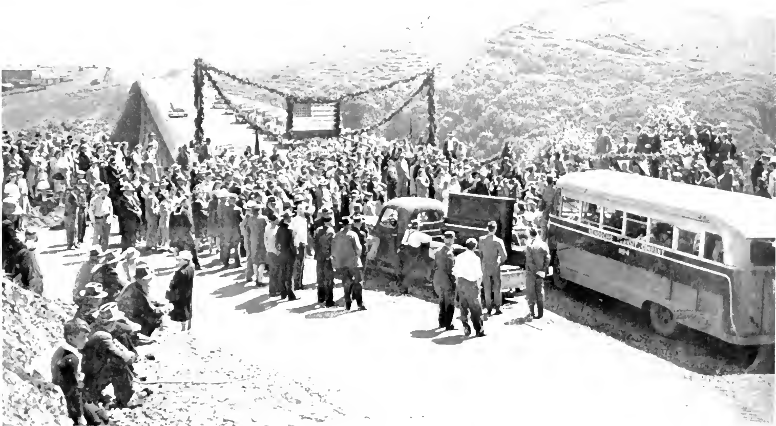
Section of crowd which attended the dedication ceremonies at the new Albion River bridge, showing speakers' platform in right foreground
